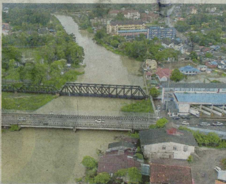
The water level in Sungai Golok has surpassed its danger mark, inundating villages in Rantau Panjang yesterday.
